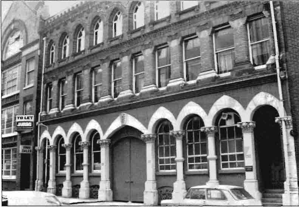
11. Former warehouse in Wellington Street, built c. 1865. Notice the cart entrance through the building which gave access to a courtyard surrounded by factory buildings of a more functional design than this elaborate façade.
