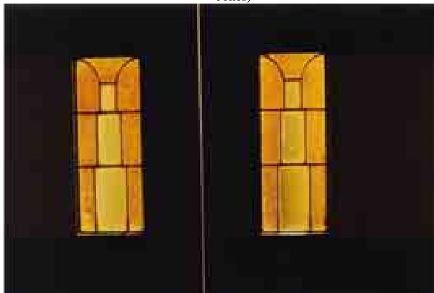
Fig. 29 Leaded lights to exit doors, main auditorium (and elsewhere)
