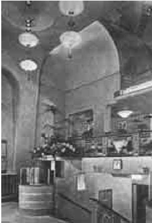
Fig. 4 Main foyer, 1936, view north-west
