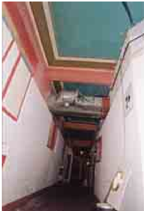
Fig. 10 Stalls foyer (50-57-27A) view south-west
