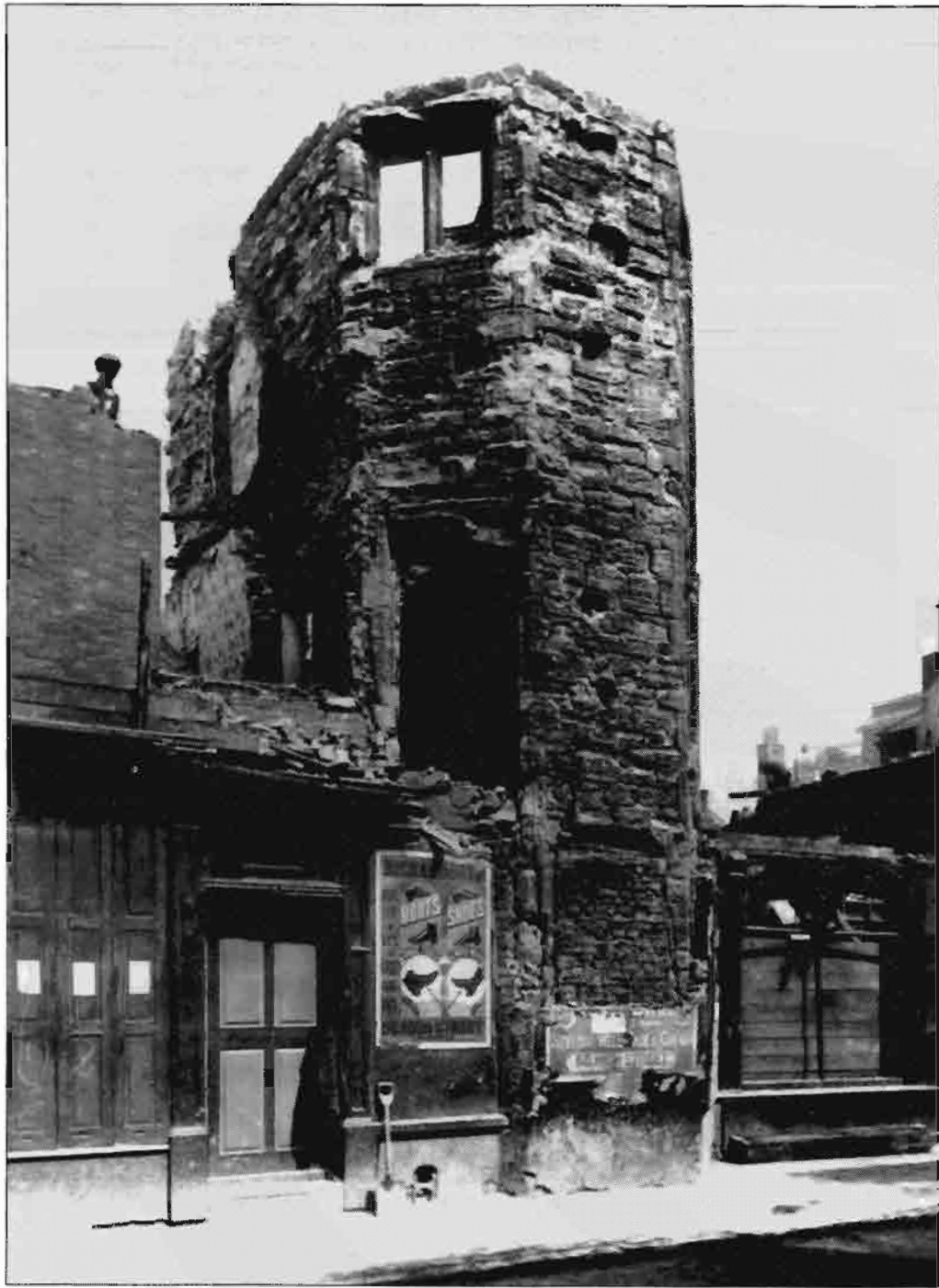
3. Tower with brick removed, during demolition in 1902
