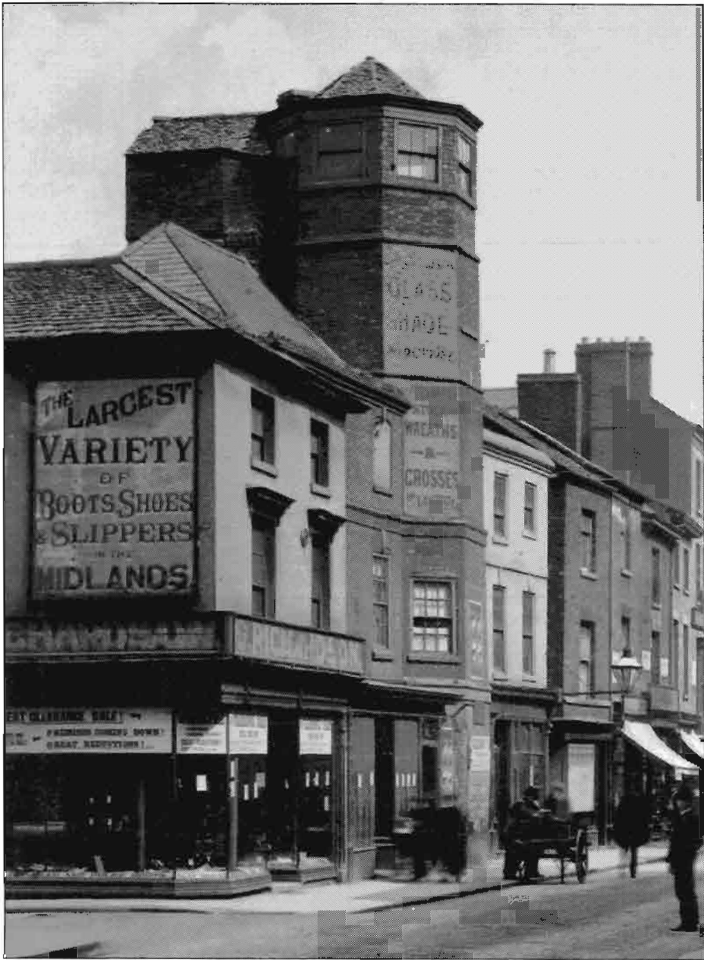
2. Tower with brick shell prior to demolition
