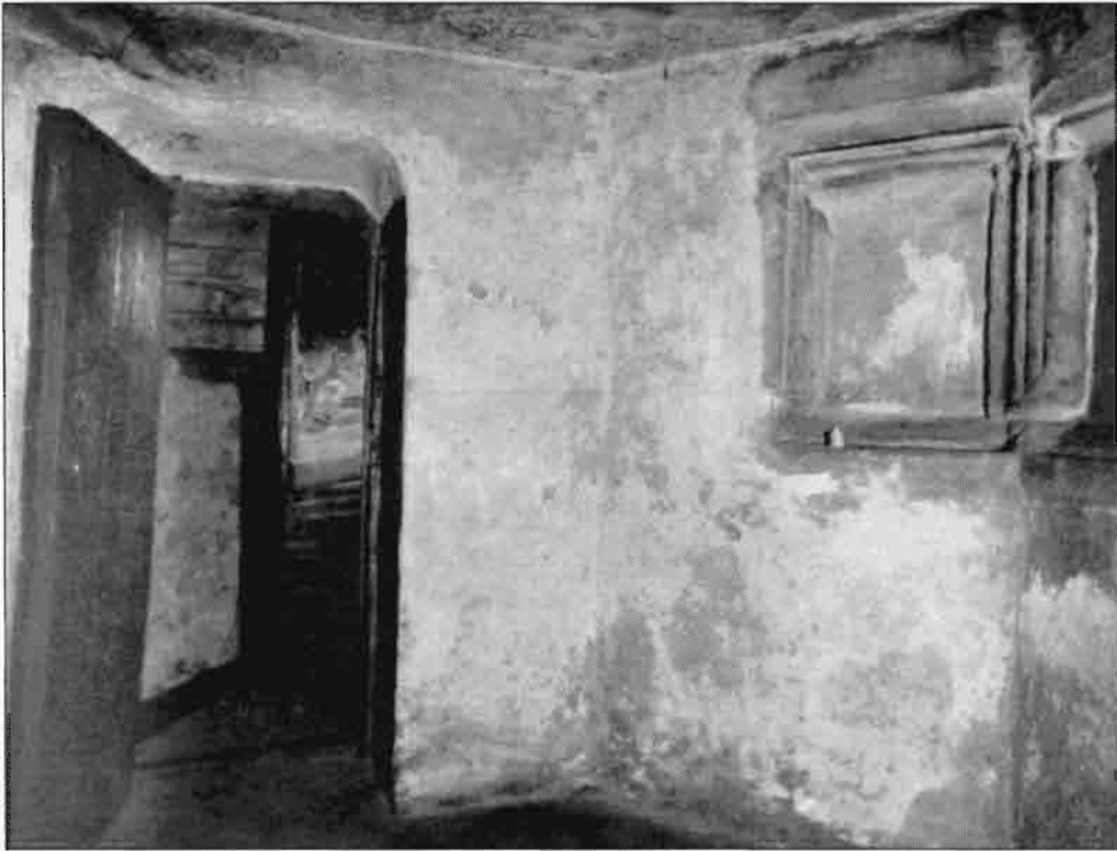
12. Inside of 3rd floor showing spiral staircase and range of blocked mullioned windows
