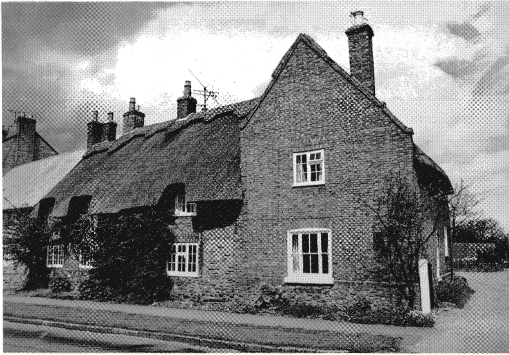
Plate 1: Hall from the street
